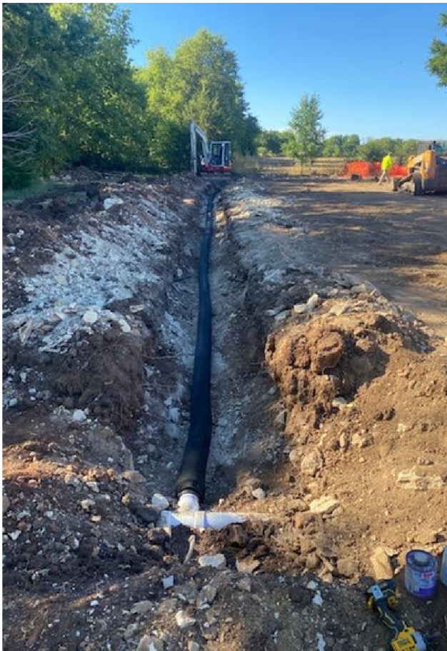
Above: flexible corrugated pipe is installed for a wastewater absorption field.
