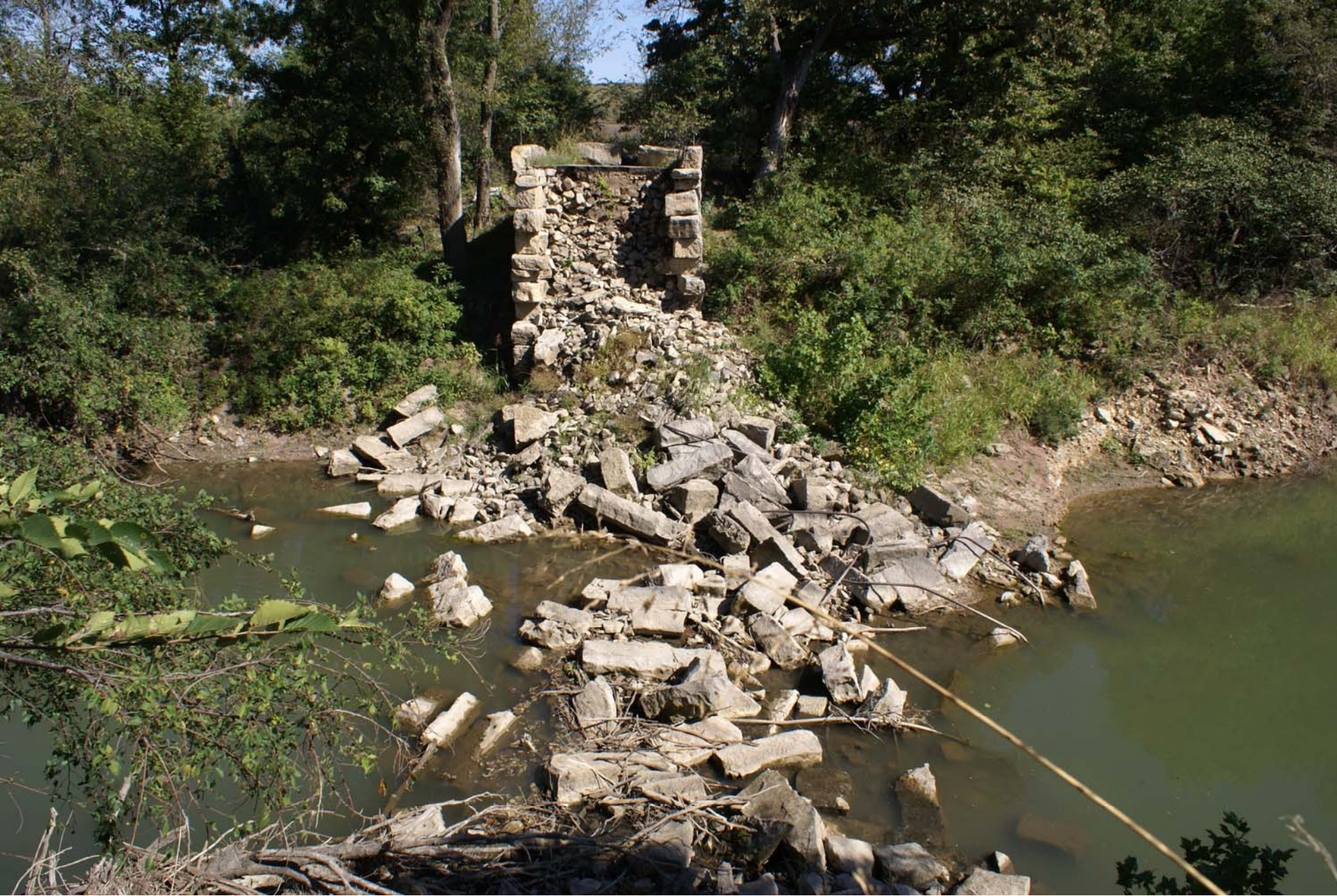
Remains of the Branson Stone Arch Bridge North of Dexter on Grouse Creek
